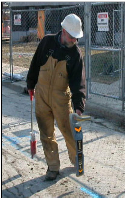
Locating buried valves and lines are no problem for ATS Techs
