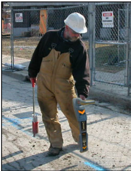
“Critical Dig” Location Specialists
