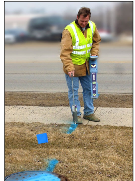
Locating buried utilities of all types is routine for ATS Technicians
