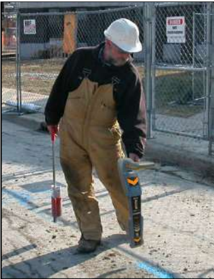
“Critical Dig” Location Specialists
