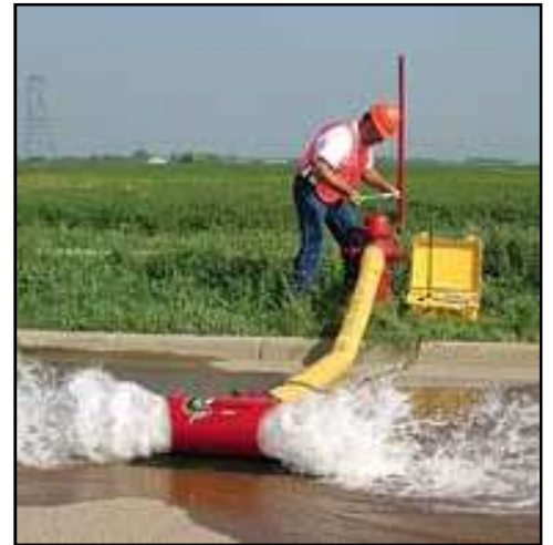
Unidirectional Water Main / Hydrant Flushing
