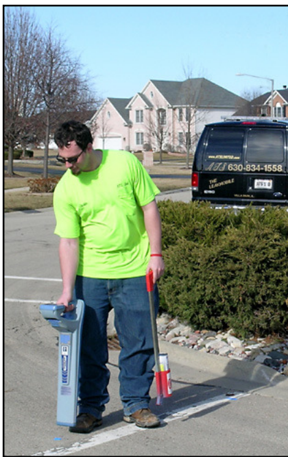
Locating buried valves is no problem for ATS Technicians
