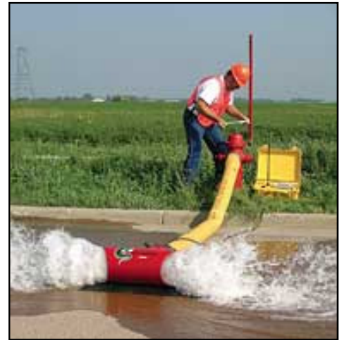
Unidirectional Water Main / Hydrant Flushing
